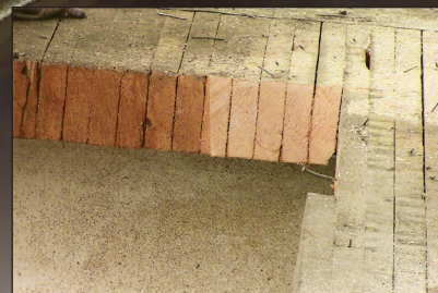
Hemlock boards standing on end formed the original factory floor
